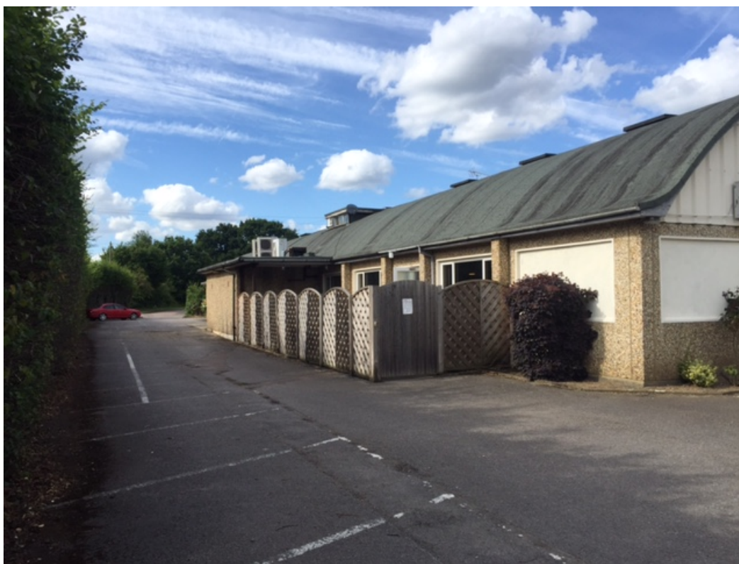
Western side of Chobham Club and hedge on boundary of Windsor Road (main road)
