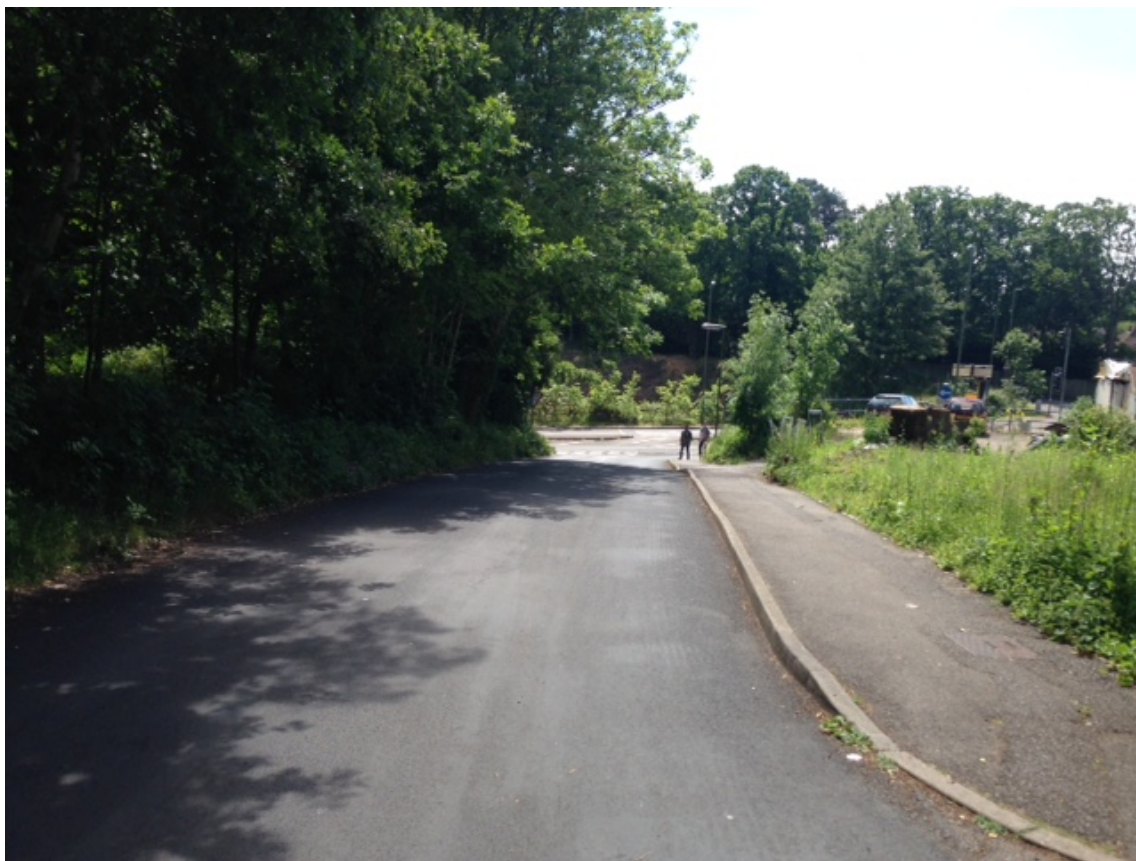
Photo showing gradient of Maultway North looking towards A30
